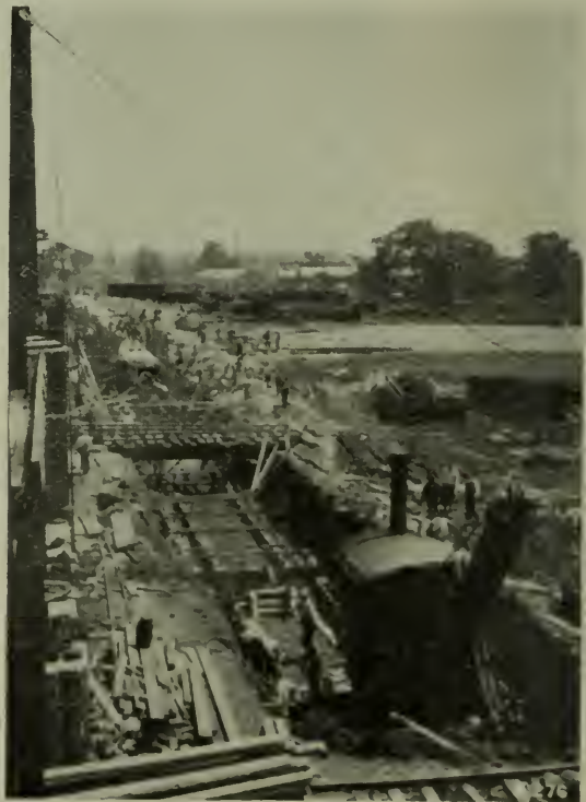
FIG. 7. STEAM SHOVEL EXCAVATING FOR SUBWAY.
